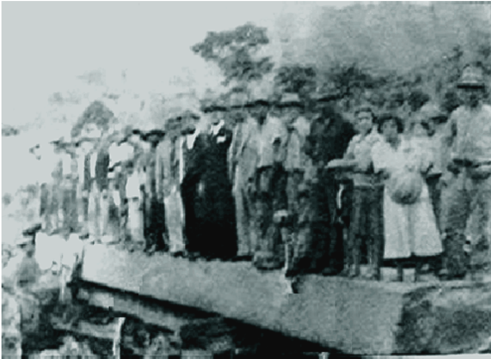
Figure 5. Piracaia black granite block with 10 m long by 1.60 m wide and 0.60 m high exploited in 1938 and his transport structure of cow car.
