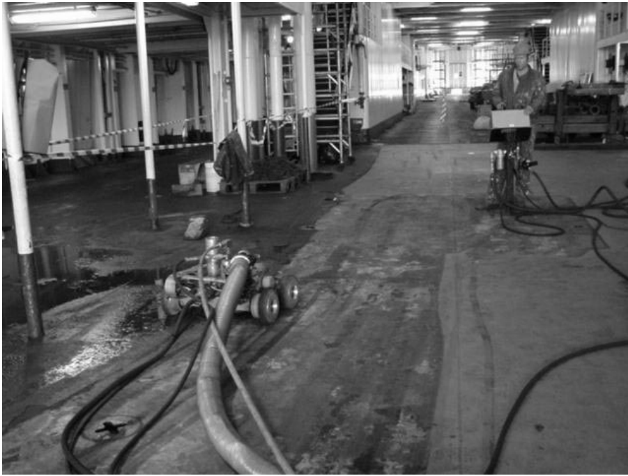
Figure 5. The original process for removing non-skid coatings from ship decks with UHP water utilized devices that were originally developed for vertical surface preparation work.
