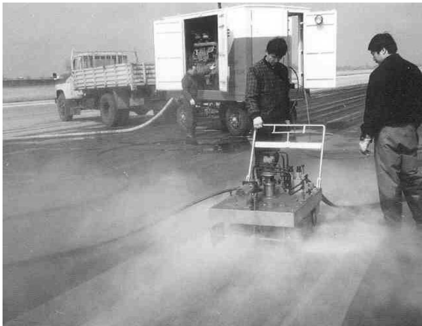
Figure 4. Testing ground of Glue Removal
