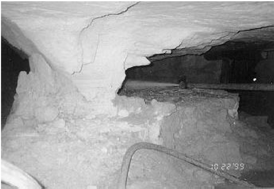
Figure 9. Roof support by leaving portion of the ore pillar.
