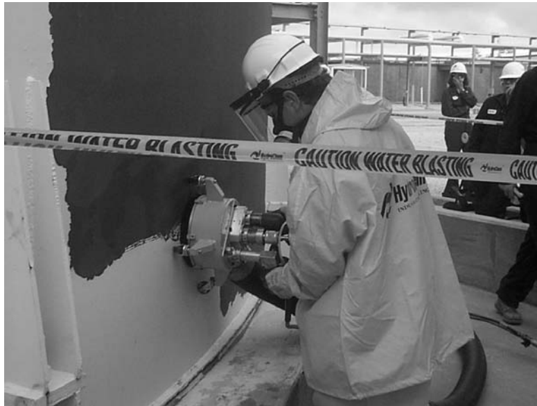
Figure 11. WJ Paint Removal with Suction
