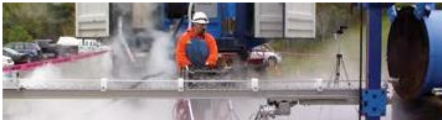
Figure 2. NitroLance can be equipped for hands free operation to provide additional safety
