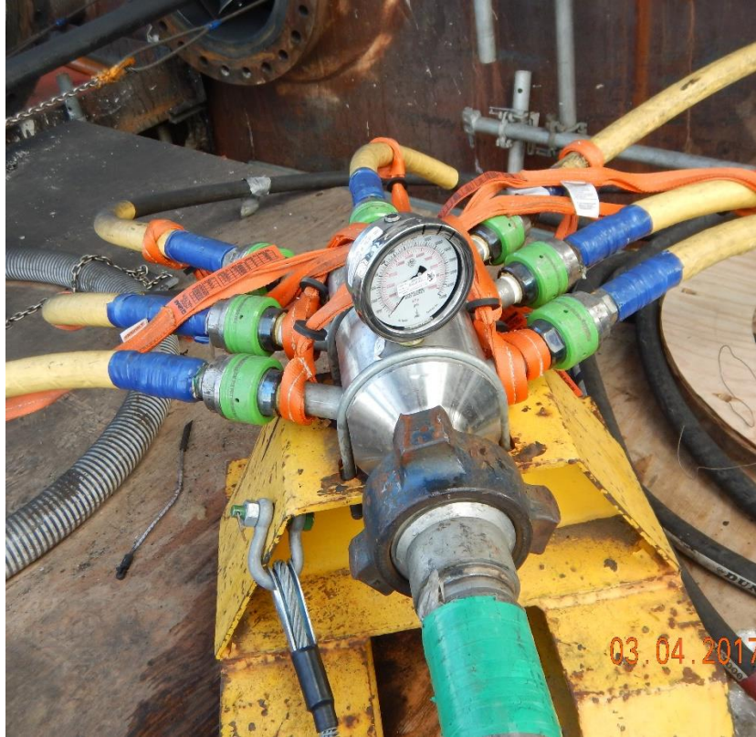
Manifold on Structure Fed by Six 1" Waterblast Hose, into Single 1-1/2" Hose Figure 1.
