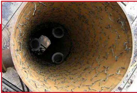
Figure 8. FCC reactor riser
