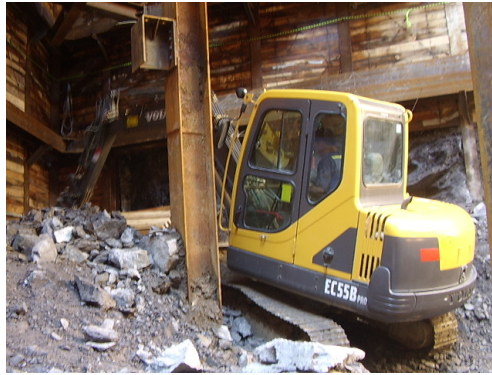
Figure 1-1 Hydraulic Breaker attacking Bottom Corner Rock under Slab Behind column
