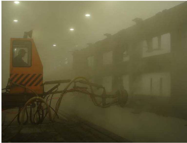
Figure 9. Underframe Rust Removal
