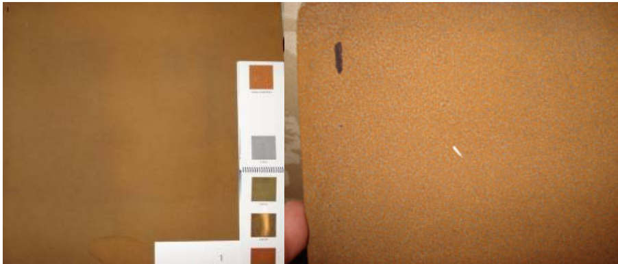
Figure 4 Moderate Flash Rust Courtesy of Ault and Cogswell, NSRP
