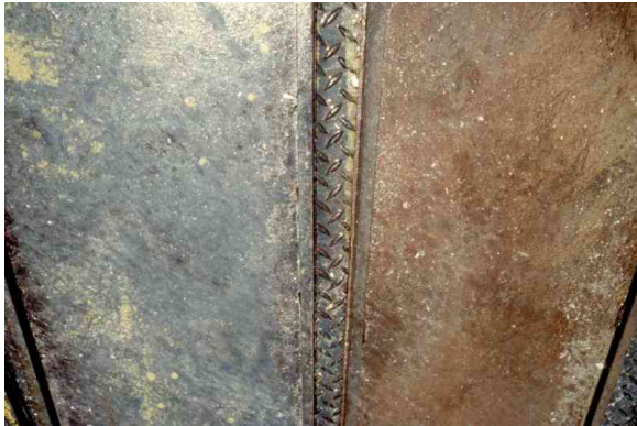
Figure 3 Initial Condition and Prior to Painting
