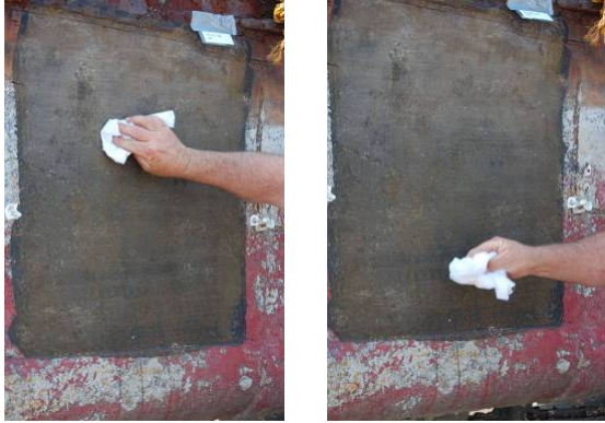
Figure 5 Cloth Wipe- Light Flash Rust Area
