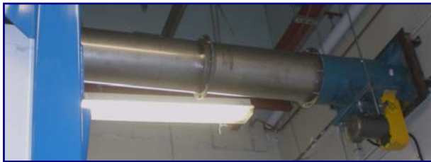
Figure 9. Close-up view of the exhaust duct from the booth.
