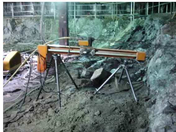
b) Tripod setup for feeding and rotation
