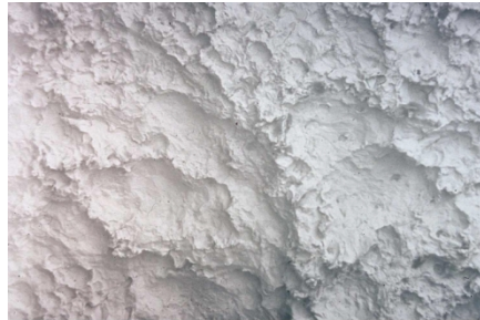
Figure 2 Water Jet Cleaned- Rounded Initial Profile
