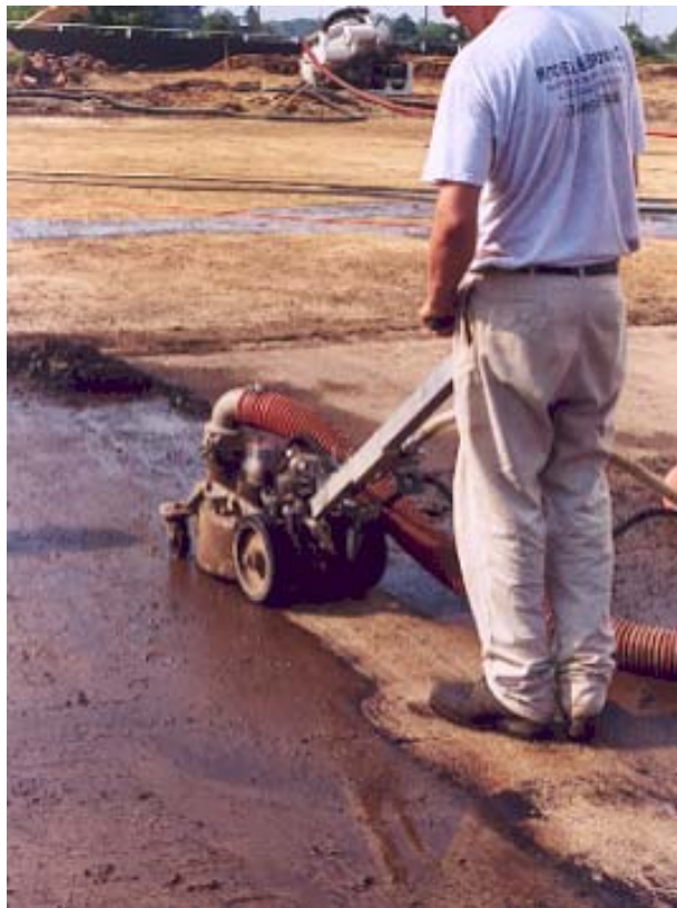
Figure 8. Membrane removal from a concrete surface.
