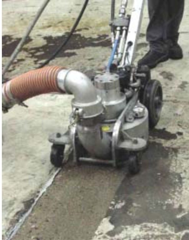
Figure 3. Semi-automated tools are the most popular for performing coating removal from concrete.
