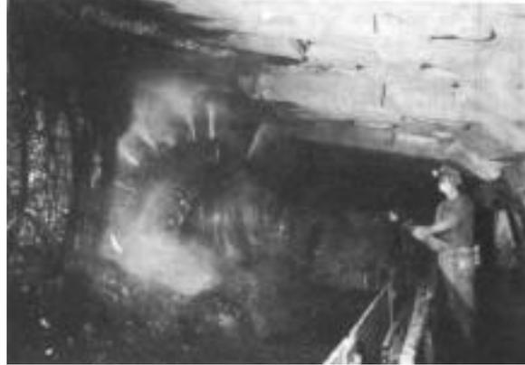
Figure 5. High-pressure water jet assistance in operation.
