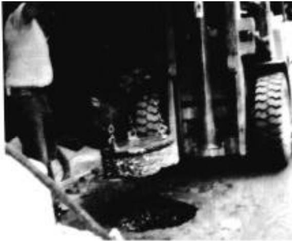
Figure 5 Removal of circular plug of pavement cut by CAVIJET nozzle.
