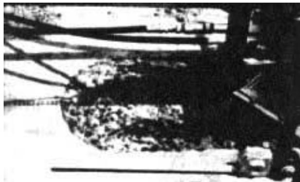
Figure 16. Light scarified concrete surface to 7 mm. Depth.
