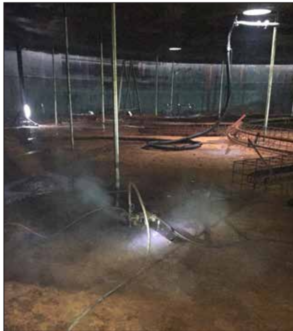
The waterjet cutting system in action. Photo courtesy Midwest Mobile Waterjet.
