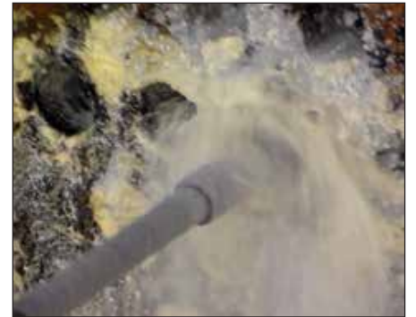
HydroDrilling a Sulfur Recovery Unit
