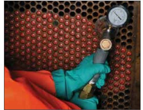
Heat Exchanger Tube Shooting
