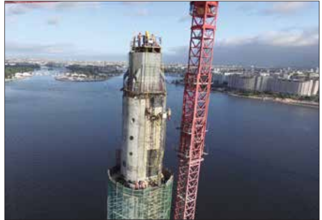
The multi-modular Aqua Spine system was chosen by ICA as being effective and flexible for this application, being assembled on the ground and lifted into position as a complete unit to further reduce set up times.
