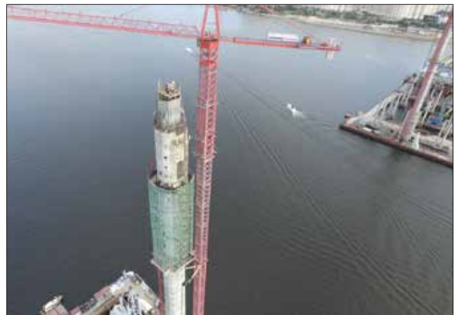
The Aqua Spine was lifted and bolted on to each side of the pylon to cover the 10 m high concrete removal area.
