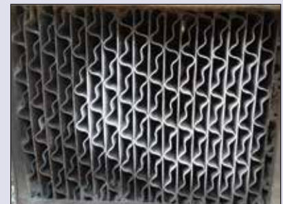
Preheater After Cleaning with NitroLance
