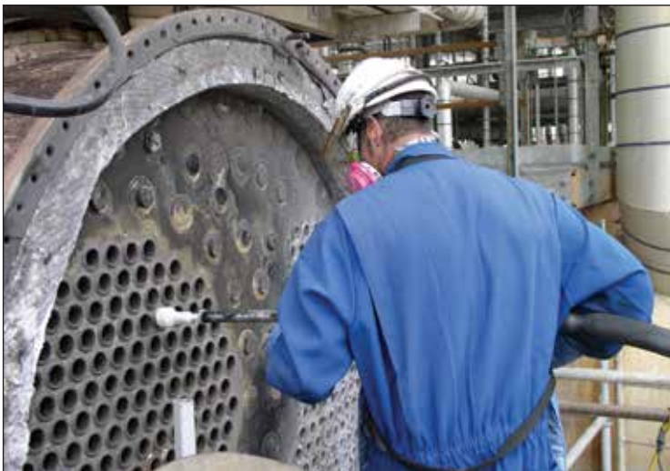
NitroLance Cleaning Tube Sheet
