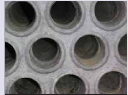
Sulfur Recovery Unit After Cleaning with NitroLance
