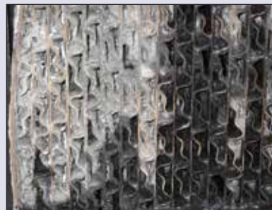
Preheater Before Cleaning with NitroLance
