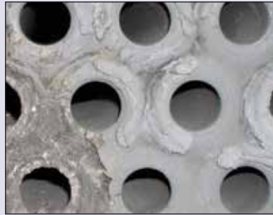
Sulfur Recovery Unit Before Cleaning with NitroLance
