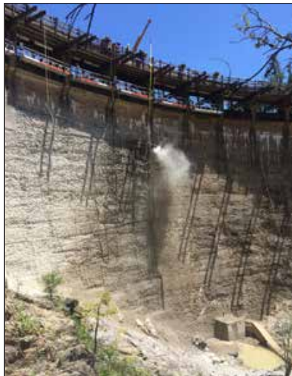
Hydrodemolition tool during water blasting sequence.
