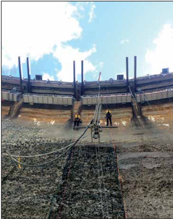
Climbers positioning and bolting robotic hydrodemolition tool to the dam face.
