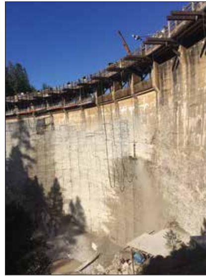
Side view showing both robotic tools - one rotary head and one oscillating head. The choice of tool was dependent on depth required and location of blasting area (crane cable interference).
