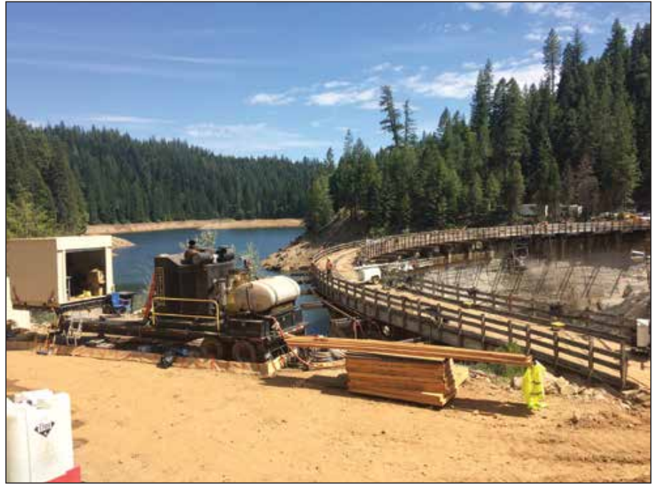
Equipment laydown areas. Three 20,000 psi pumps and water system (not shown) were set up in a very confined space.
