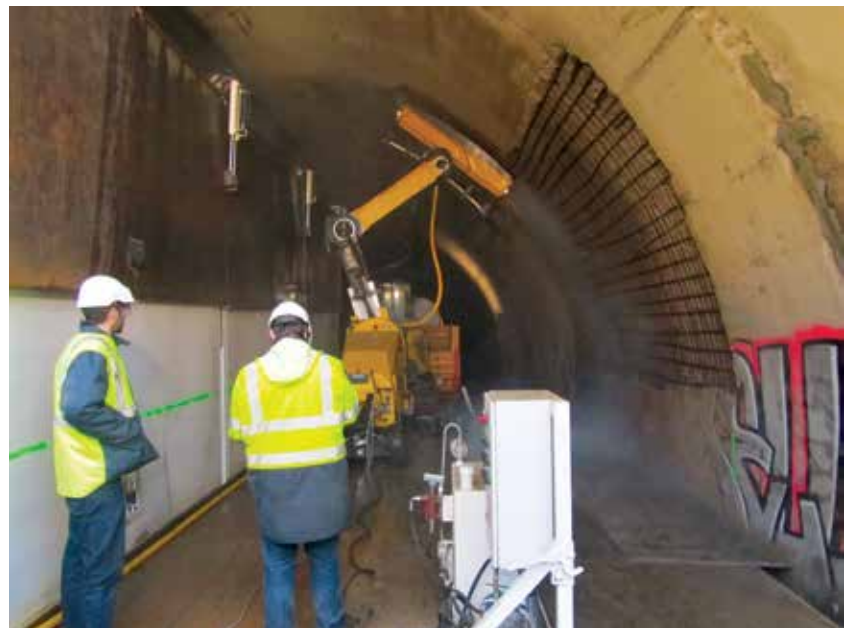
Hydrodemolition with a Conjet Robot 365 was used to selectively remove the damaged and decaying concrete at record speed from the Biéreau Tunnel just south of Brussels.
