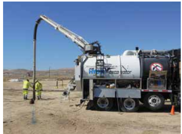
Hydro-excavation uses high pressure water to loosen soils, and the residual slurry spoils are easily extracted into the debris tank via a positive displacement blower or centrifugal compressors.
