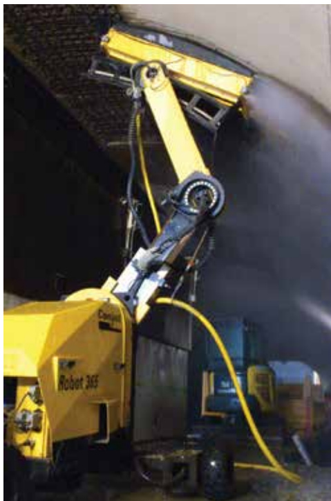
Hydrodemolition with a Conjet Robot 365 was used to selectively remove the damaged and decaying concrete at record speed from the Biéreau Tunnel just south of Brussels.
