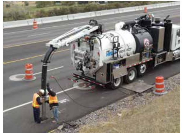
The key to efficient hydro-excavation is to use the proper amount of water for the job. This will maximize productivity and operator efficiency.
