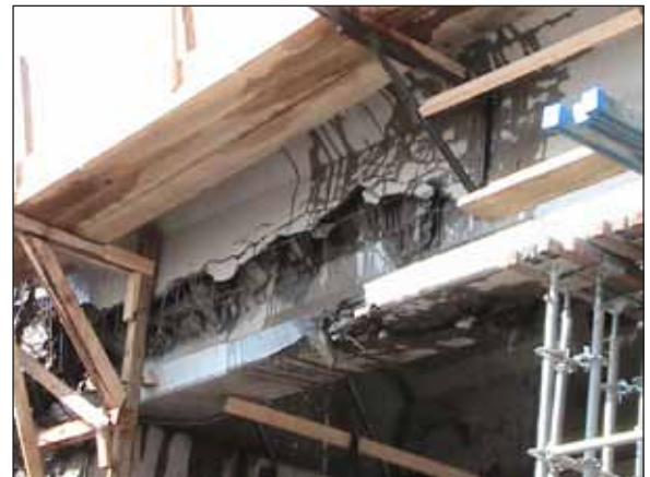
Badly damaged concrete beams on two bridges in Chile, caused by an earthquake were removed using hydrodemolition techniques. This proved ideal with no collateral damage to the remaining structures.
