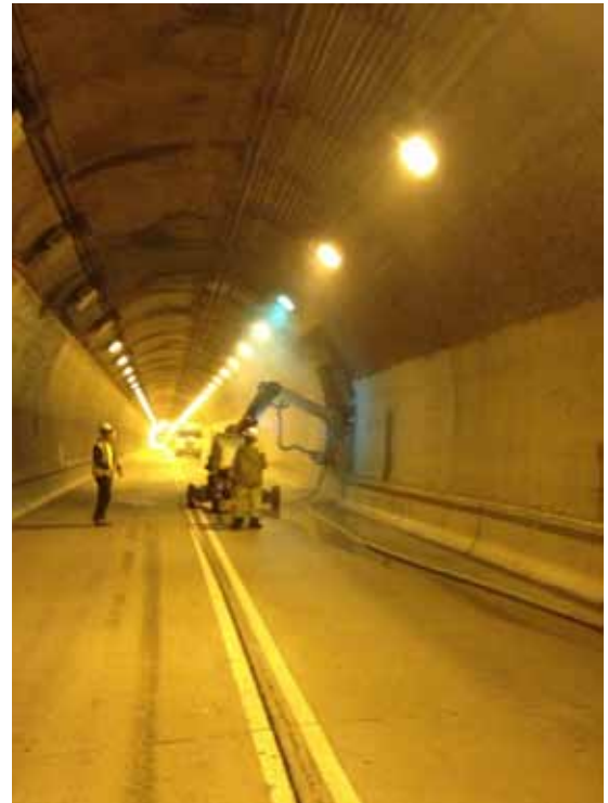
Two Conjet Robot 363 hydrodemolition machines have been adapted to suit the curvature of the horseshoe shaped walls of the two Liberty Tunnels. See article, page 2.
