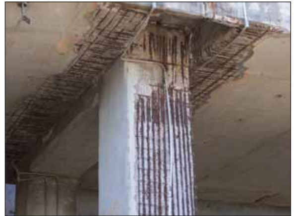
Typical heavy concrete damage to an elevated concrete decking.
