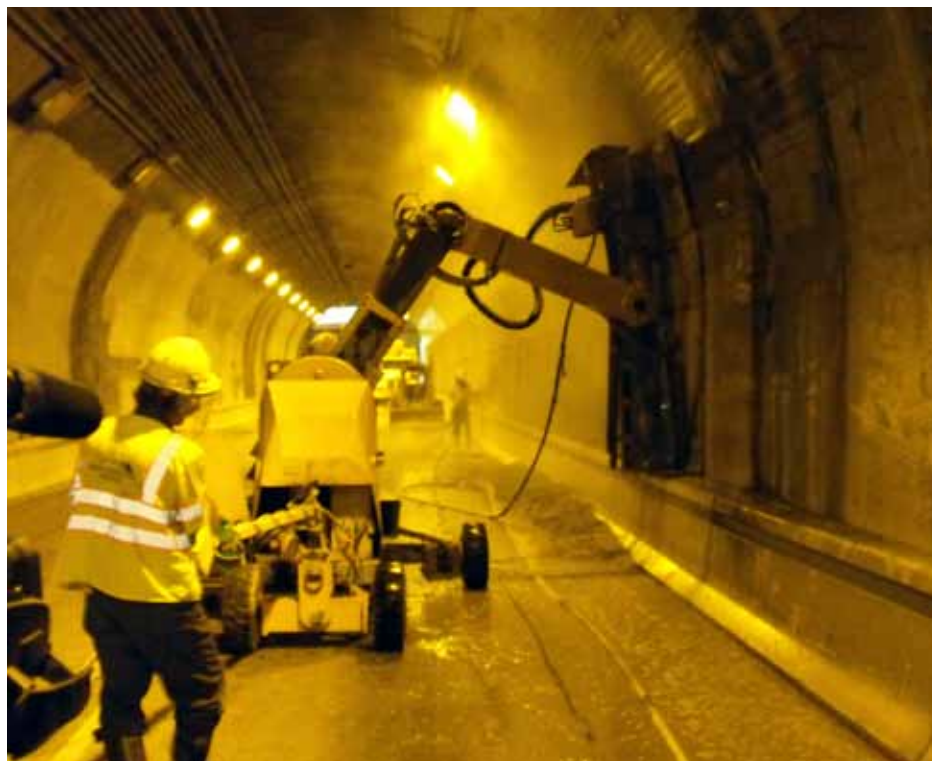
The Conjet Robot 363 adapted to suit the curvature of the horseshoe shaped walls.
