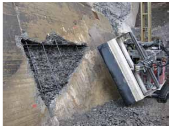
A basic principle of hydrodemolition is ‘selective removal’ - removing only the amount of concrete needed for the refurbishment and leaving ‘good concrete’ and steel reinforcement undamaged.
