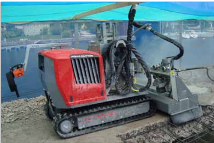
Hydrodemolition techniques offer a fast and efficient method of concrete removal, without damaging the surrounding structure and imbedded rebar, utilizing power from high-pressure water.
