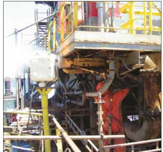
Waterjetting being used for essential corrosion prevention maintenance on the rig structure.
