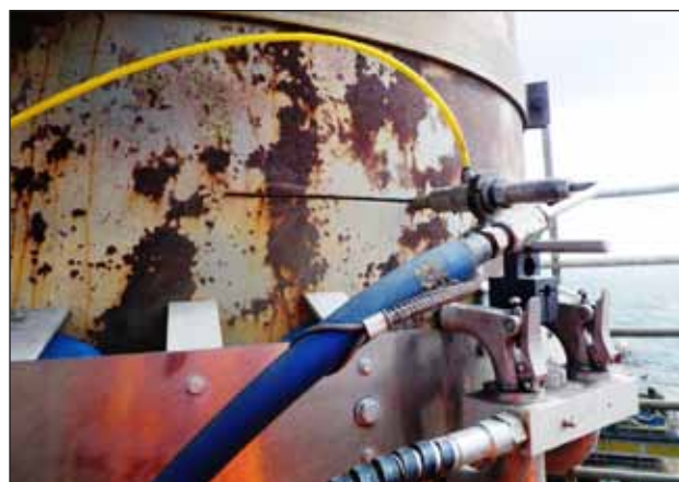
Jet Edge Spyder package making initial cut on contactor tower.
