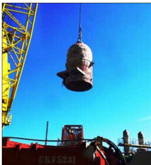
Contactor tower top section after successful waterjet cut - note two remaining towers in background.
