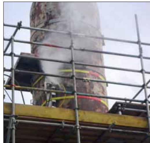
Vertical cut in progress for “mailbox” internal inspection window.
