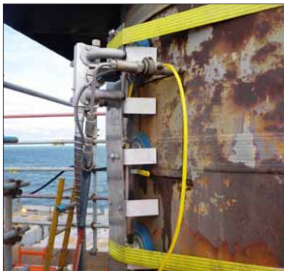
Jet Edge Spyder set up on rigid track for vertical cut.
