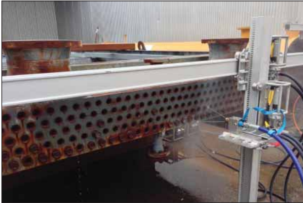
Flexframe attached to the headerbox of an Airfin cooler with rotating gun nozzle.
