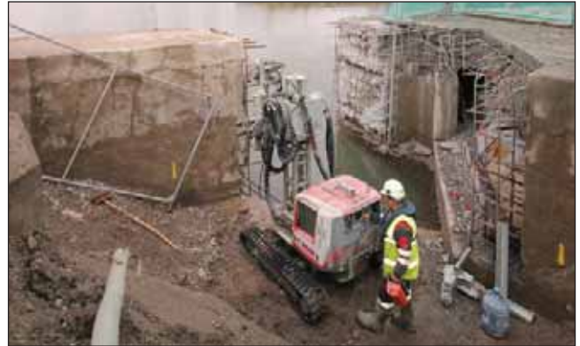
Hydrodemolition was carried out without disrupting shipping movements to adjacent quays.
