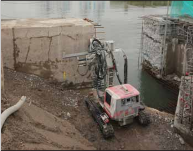
Robotic hydrodemolition duties were initiated on completion of wiresawing the concrete face to expose the rebar.
