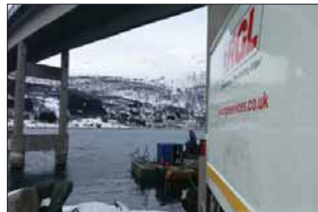
A unifloat barge and crane was supplied by Multibetong for positioning the hydrodemolition equipment alongside the bridges columns.
