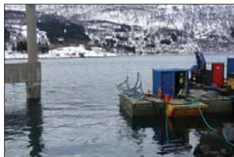
The pontoon was used to house the containerized hydrodemolition robot and power pack, the column blasting rig and a generating set. A shore-based truck mounted waterjetting unit provided water via high pressure hoses.
