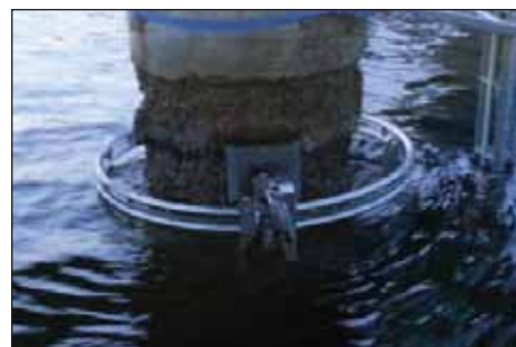
The column blasting rig was operating in sea water to depths of 20 m and temperatures below 4°C.
