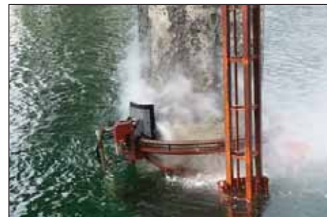
The hydrodemolition robot and Aqua Spine system was operated remotely on board the unifloat barge.
