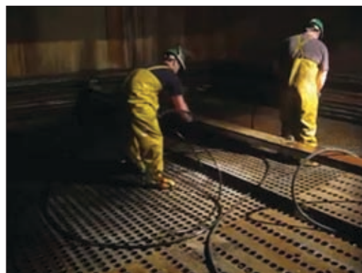
Manual lancing of vertical tubes.
