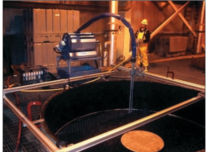
Automated lancing of vertical tubes with the SRT-100.
