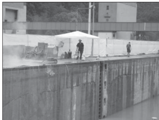
The lightweight Aqua Cutter was chosen to meet critical weight loadings in order to prevent the badly cracked lock wall from collapsing.
