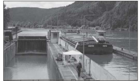
Traffic is able to use one lock while Luckei uses the Aqua Cutter to remove 400mm of concrete along the full length of the 100m long wall.
