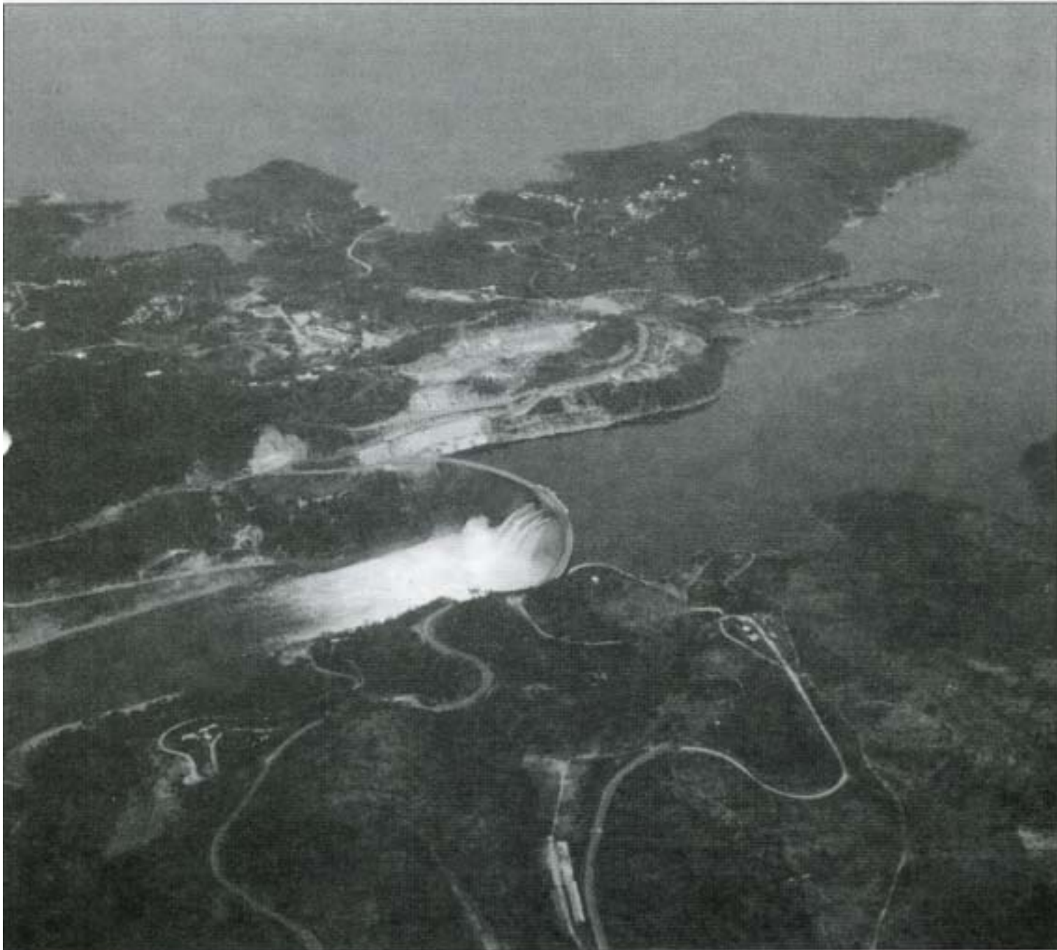
Water jets issuing from sluice gates in the Kariba Dam on the Zambezi River in Africa. Photograph reproduced by permission of Garrett Educational Corporation, Ada, OK , from How We Build Dams by Neal Ardley.
