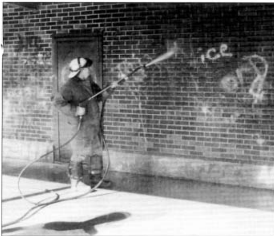
Donald J. Huber, Supervisor for the City of Alton, Illinois, removes gang graffiti from a building in Salu Park in Alton. See "Water Jets Erase Gang's Signs" on page 4 of the June/July 1996 Jet News . Photograph courtesy of Russ Smith of the Alton Telegraph .
