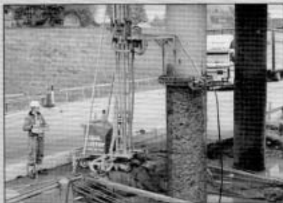
Circular powerhead on bridge deck columns.
