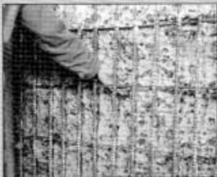
A wall in which concrete around rebar has been removed.
