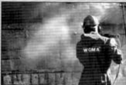
Exposing reinforcement bars with the ECOTHERM® 500 and rotating carrier head.
