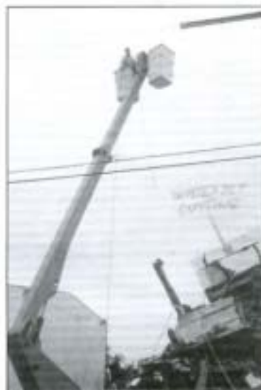
Figure 1. Superjet cutting concrete during rescue efforts in Guaratuba, Brazil. The concrete walls were cut with a 26,000 psi, 7 gallons per minute waterjet.
