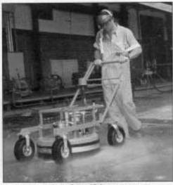
A demonstration of scarifying a concrete surface by StoneAge, Inc.
