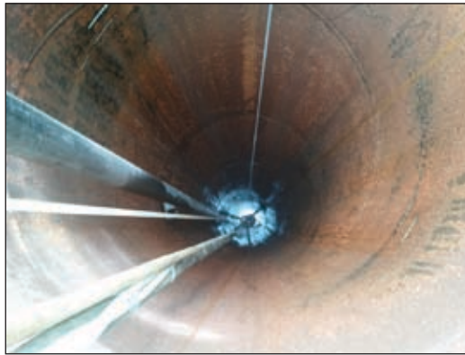
Midwest Mobile Waterjet designed and built a waterjet cutting tool that was used to cut out piles from a temporary work pier at the John James Audubon Bridge construction site in Louisiana. The cutting tool was lowered down the inside of the piles and cut them at the required depth.
