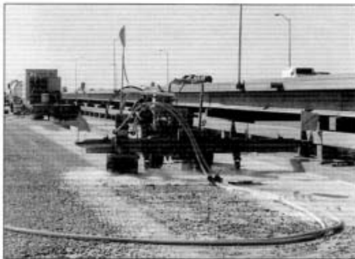
To prepare the bridge deck for a 2-1/2-inch overlay, the contractor used a hydrodemolition robot to remove a 13-1/2-foot-wide lane to a nominal depth of 1/2 inch. Photo courtesy of Blasters, Inc.
