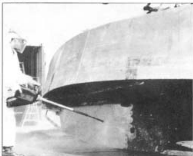
Dust free coatings removal on aluminum without costly metal removal.
