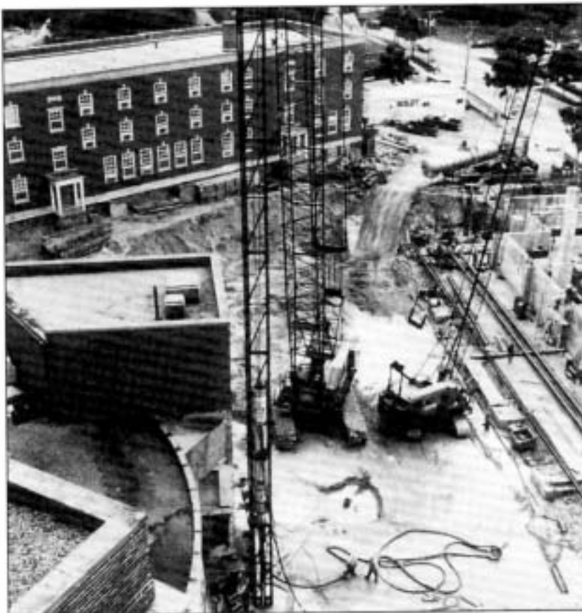
Boldt personnel use two cranes to implement an innovative waterjetting technique to drive 140-foot H-piles at St. Marys Hospital Center jobsite in Madison, Wisconsin. The technique solved structural damage and soil problems the team experienced while using conventional pile driving
