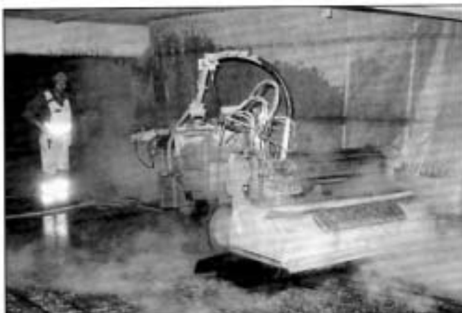
A Conjet Robot high pressure water jetting hydrodemolition machine repairing a damaged multi-story carpark at the head office of Sweden's telecommunications giant Ericsson.
