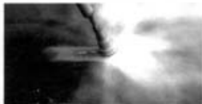
White metal finish left on steel.
