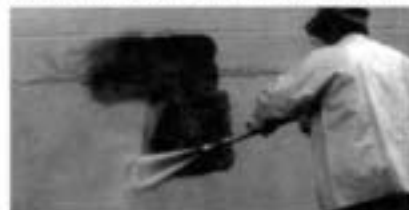
Paint easily removed from cement.
