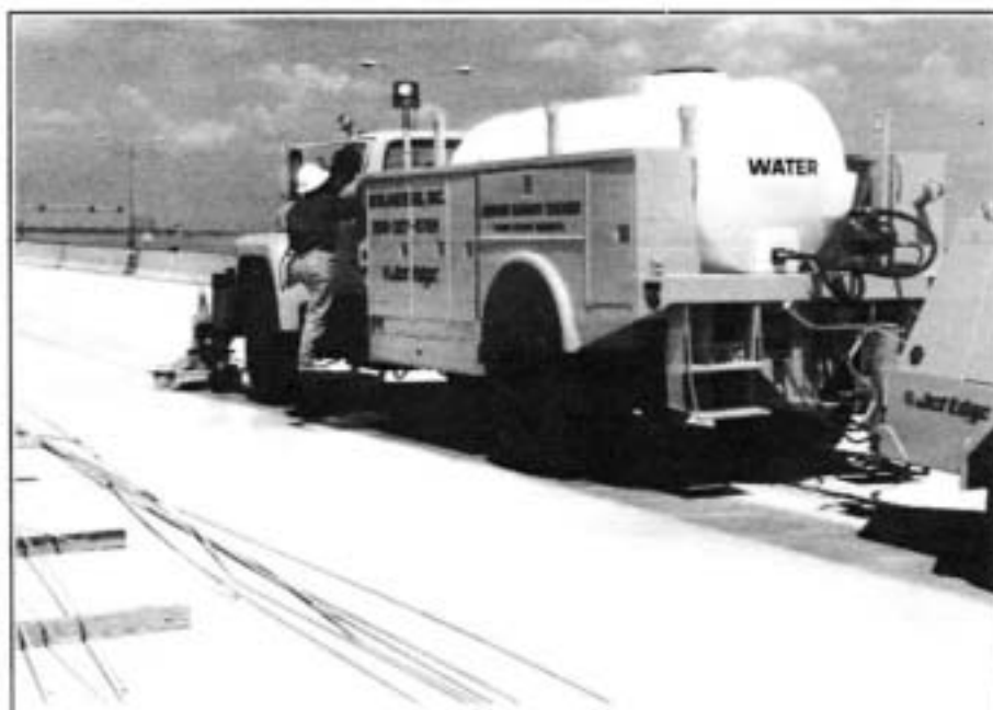
Airport runway cleaner stripping a film off a bridge. Photo courtesy of Jet Edge.
