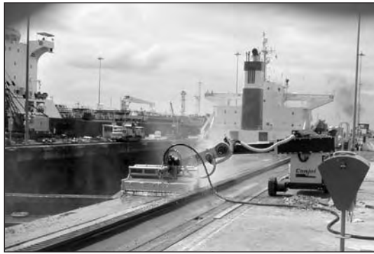
Conjet hydrodemolition equipment selectively removes weakened and damaged concrete from numerous structures, such as the Panama Canal locks.
