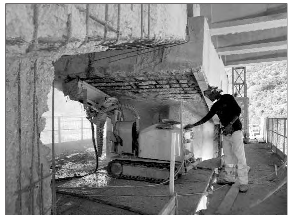
The main focus of the hydrodemolition repair with the Conjet 322 Robot is on the octagonal shaped piers and their crossheads, where the de-icing salt has leaked down from the deck above.
