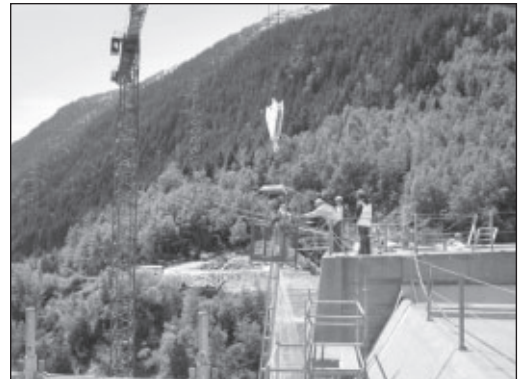
The 11-meter tower being lifted in place.
