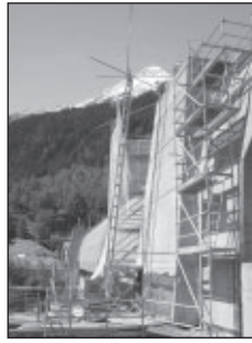
The robot tower was installed to match the 10° inclination of the tunnel wall.
