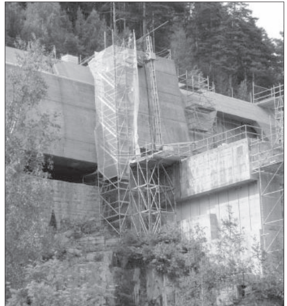
The Aquacutter 6m standard tower was extended with an additional 5.5m tower element to reach a maximum height of 11.5m.
