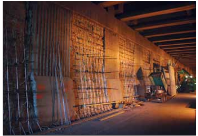
Additional rebar was installed before the new concrete.
