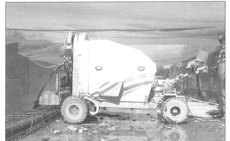
E-Schakt's Conjet Robot 362 removed the concrete from the bridge parapets leaving the reinforcement and services intact, ready for more rebar and new cast in-situ concrete edge beams. Photo courtesy of Conjet AB.
