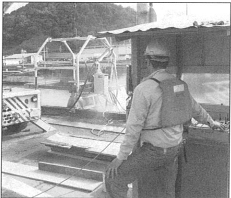
The computer-controlled Conjet Jetframe hydrodemolition equipment is remotely operated.
