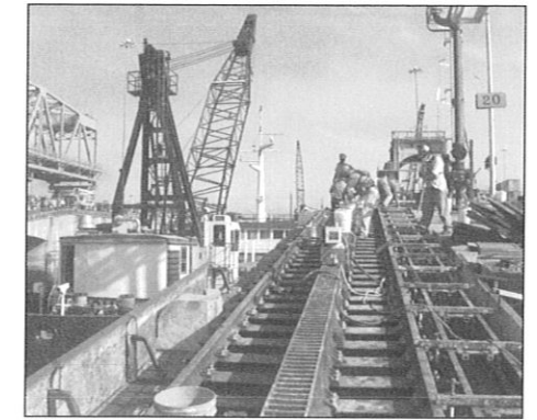
Installing new sections of prefabricated tow track along the tops of the locks.
