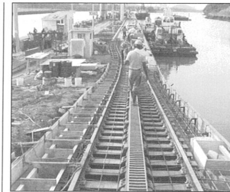
Installing new sections of prefabricated tow track along the tops of the locks.
