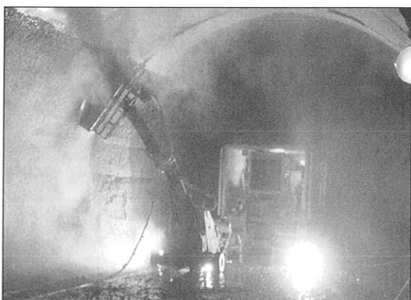
CO.I.P.I.'s Conjet Robot 362s assisted in high speed tunnel repairs at Bolzano in Northern Italy
