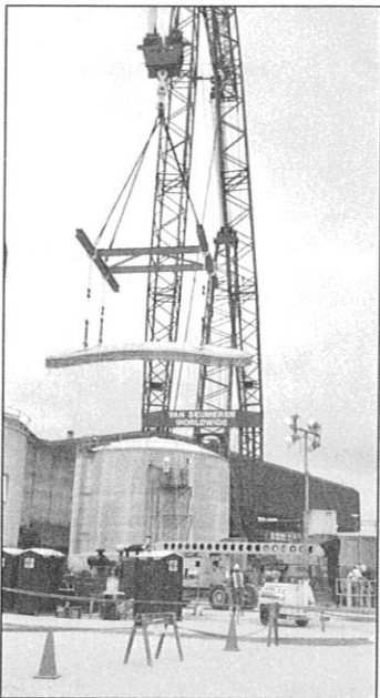
An oval of reinforced concrete approximately 45 feet in diameter and 24 inches thick suspended on a 200,000-ton capacity crane. The picture above shows the concrete oval just lifted from the dome. The picture on the right shows the concrete oval being lowered. The oval of reinforced concrete weighed 160 tons. This high capacity crane was used to provide a large factor of safety during lifting. This crane is one of the largest in existence. It used four million pounds of counterweight and arrived on site in 157 tractor-trailers. Photographs reprinted courtesy of North American Services Group.
