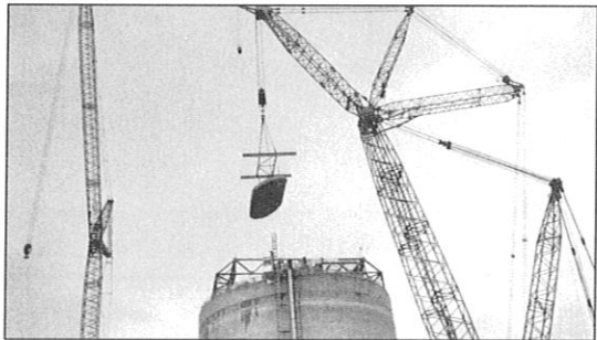
An oval of reinforced concrete approximately 45 feet in diameter and 24 inches thick suspended on a 200,000-ton capacity crane. The picture above shows the concrete oval just lifted from the dome. The picture on the right shows the concrete oval being lowered. The oval of reinforced concrete weighed 160 tons. This high capacity crane was used to provide a large factor of safety during lifting. This crane is one of the largest in existence. It used four million pounds of counterweight and arrived on site in 157 tractor-trailers. Photographs reprinted courtesy of North American Services Group.
