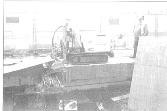
Contractor Mowlem is using Doornbos Rental UK's Conjet Robot 322 in Plymouth to remove concrete from the viaduct deck and finger beams to expose the reinforcing ready for casting on an extension to the deck.
