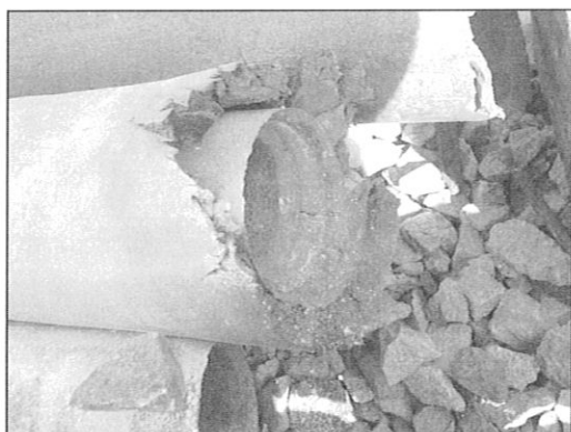
Cut-off insulated pipe. Black rubber insulation shown on the outside of a four-inch pipe. Three-inch pipe shown inside of four-inch pipe. The presence of the rubber insulation ruled out the use of thermal cutters on this job. Waterjet cutting being a cold-cutting method was the superior choice for this application.
