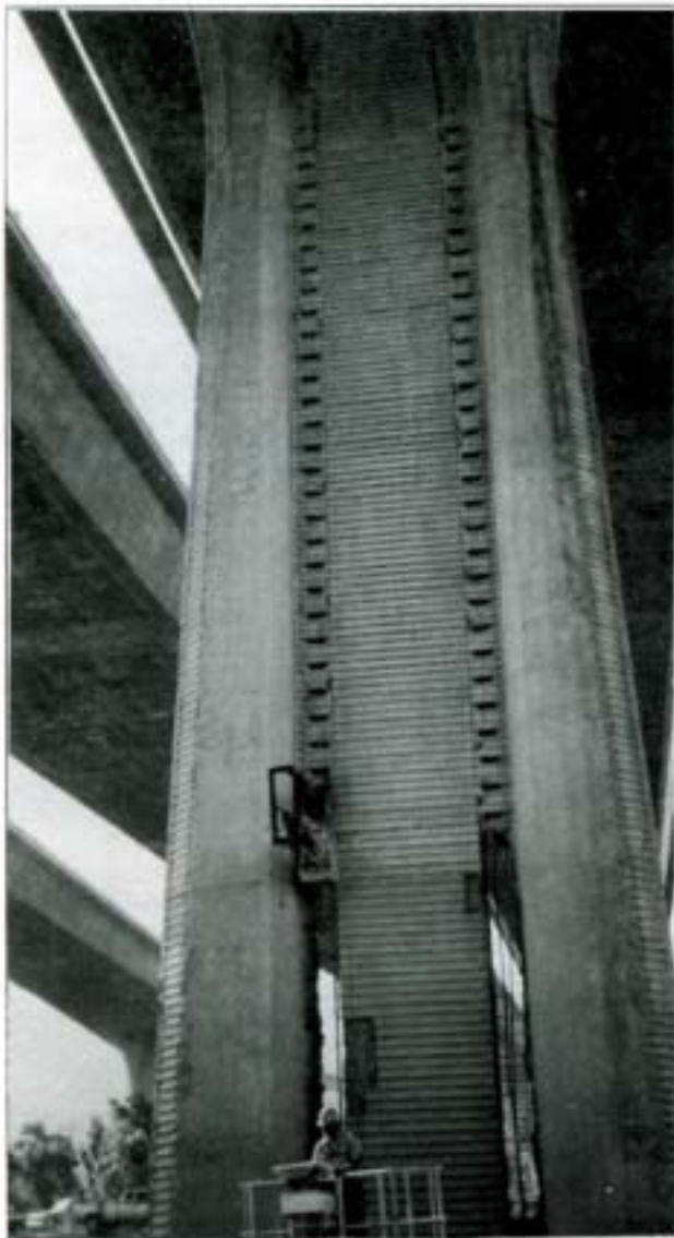
This photo shows the abrasive jet drill on a pillar.
