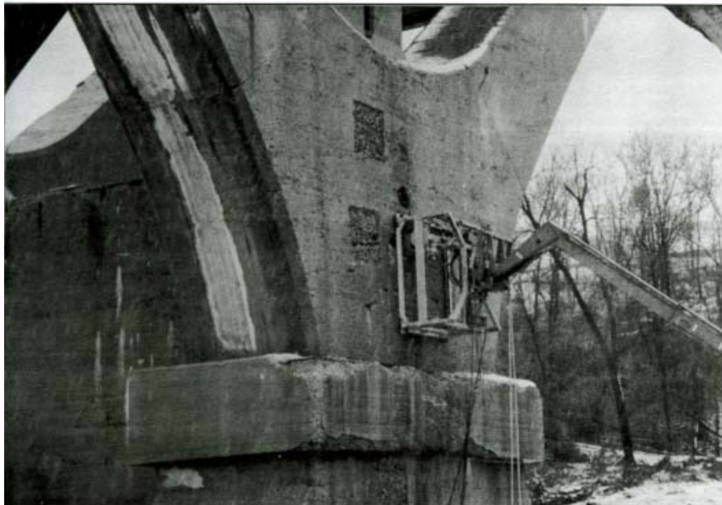
Rotating water jets (36,000 psi), mounted on the computer guided carriage of the Porta Blaster, blasts away unsound material from concrete arch. Photograph courtesy of Jet Edge, Inc, Minneapolis, Minnesota.
