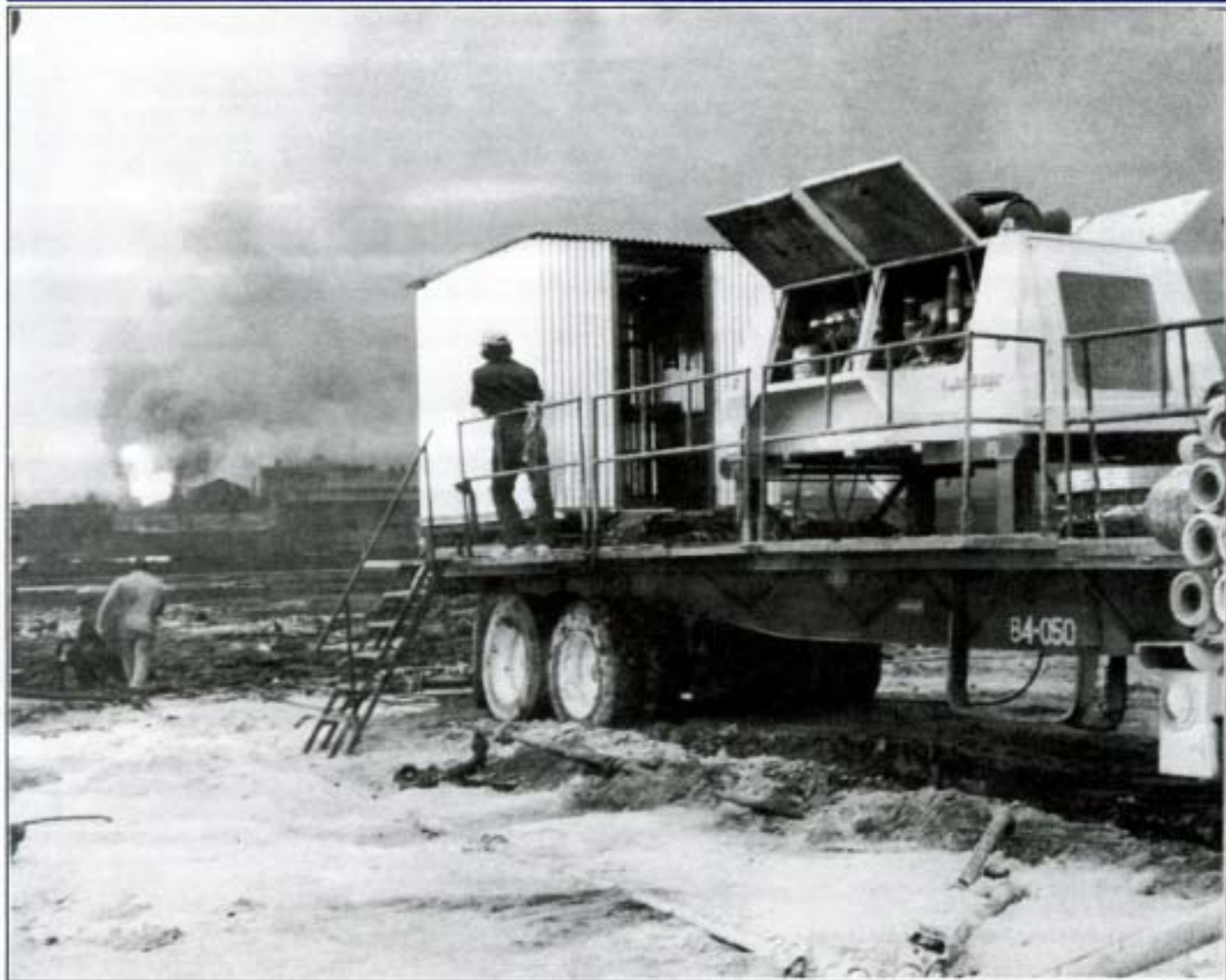
A water jetting worksite in a burning Kuwaiti oil field.
