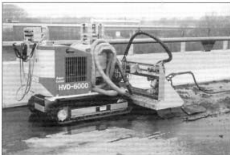
Aqua Cutter Hydrodemolition Robot. Photo courtesy of Aquajet Systems AB.
