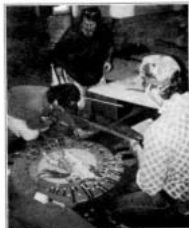
Crossville Ceramics artistic advisor David Wright oversees the installation of the water jet cut pieces of porcelain tile that form the Wildhorse logo. Each piece was numbered and covered front and back with clear contact plastic. The installer peels the back plastic, and sets the piece with the front plastic still in place.
