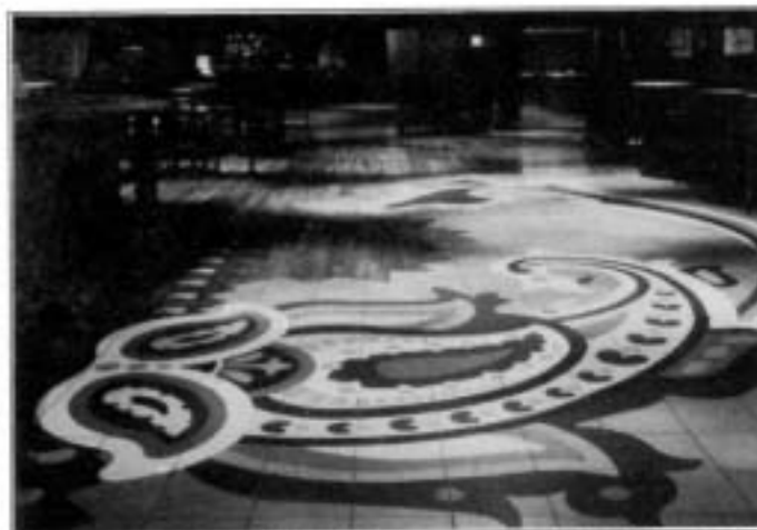
Sized to suit a giant, the bandanna covers nearly 1,000 sq. ft. of floor space, making it one of the largest tile installations to use a water jet design since Crossville introduced the program.
