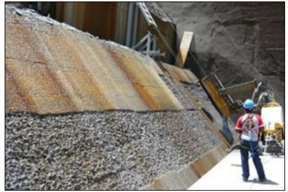
The Conjet Robot 364 selectively removed the weakened and damaged concrete from the spillway surfaces to depths ranging from 20 mm to 150 mm and in some instances exposing the steel reinforcement.
