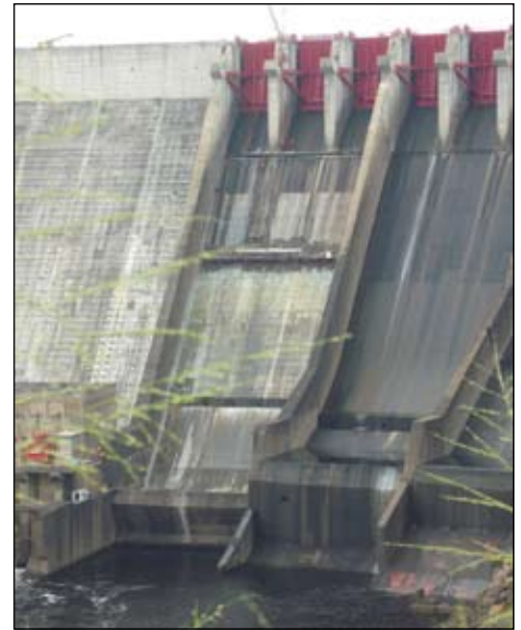
Fapco's purpose built working platform was moved up and down the steep spillway channels by four winches mounted on the crest of the dam.
