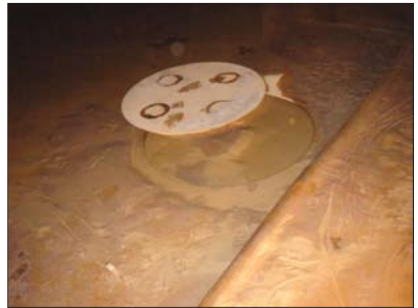
Gasoline tank cut with an abrasive jet.
