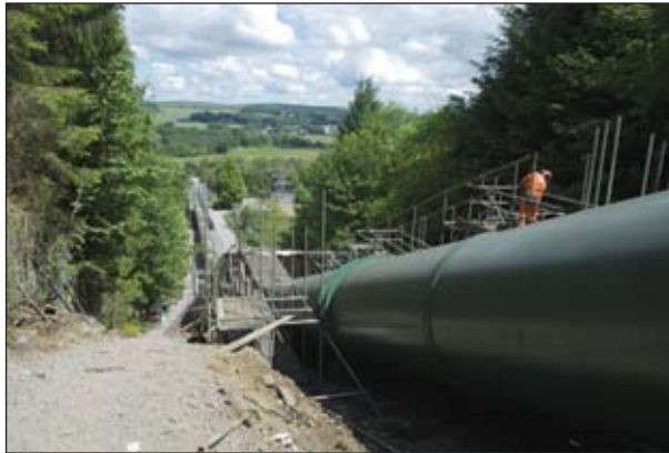
Water plunges 125m down the hillside through a 570m long steel penstock of varying diameter to Glenlee power station's twin 6MW turbines.
