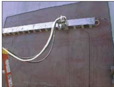
AK Services uses waterjets to cut accesses into storage tanks.
