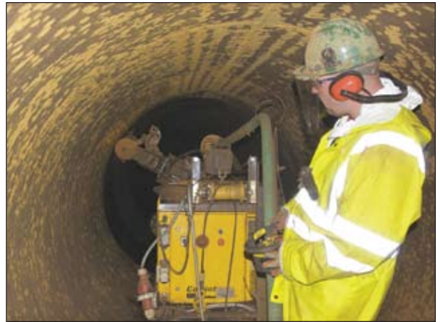
N.E.T. had to clean about 4,200m 2 from the inner surface of the 1.8m to 3m diameter penstock with its Conjet 324 Robot working on gradients up to 18°.
