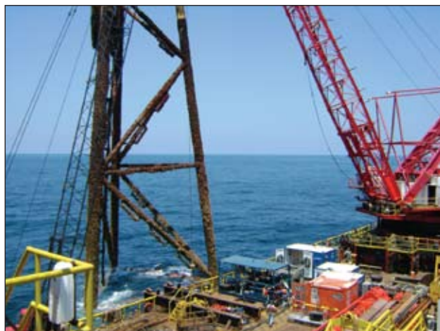
Proserv Offshore's Subsea & Marine Technology division, based in Houma, La., uses waterblasting equipment along with abrasive to help dismantle offshore platforms and wells.
